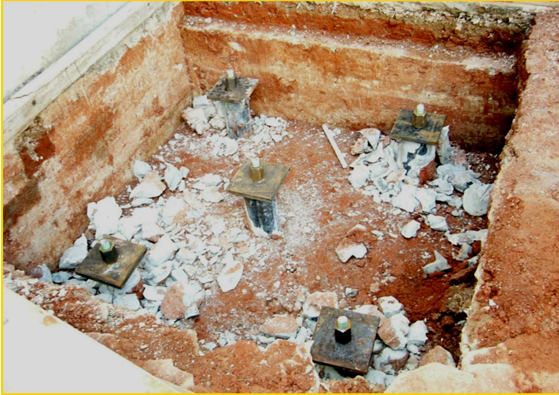
Figure 10: Micropile Pile Cap Excavation Showing Bar Piles with Top Pipe Reinforcement
